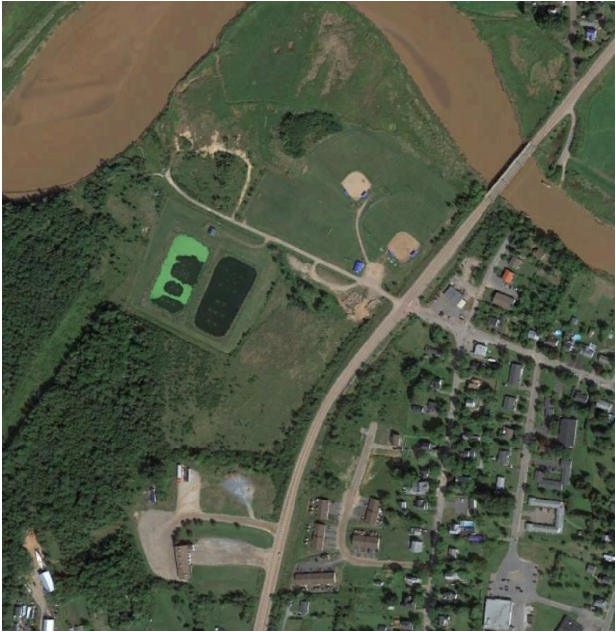
Figure 5-6: Stewiacke Wastewater Treatment Plant
