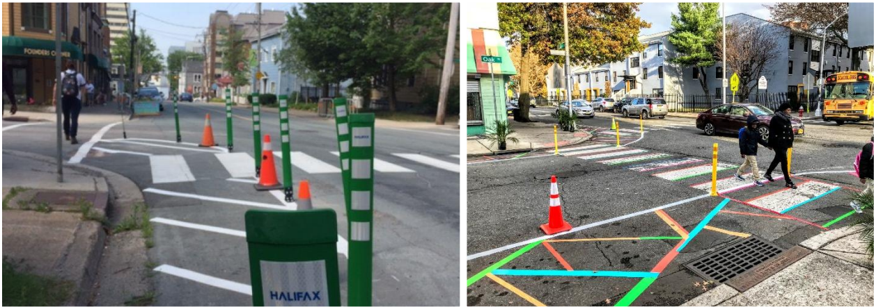
Figure 7-18: Example – Use of Removable Bollards and Paint
