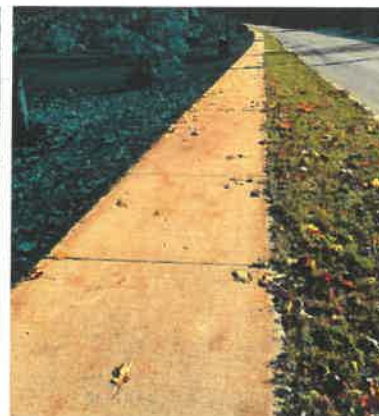
Concrete paving with even surface
