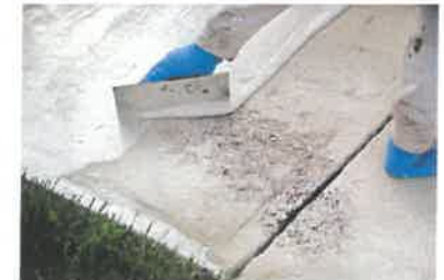
Concrete overlay/ Resurfacing
