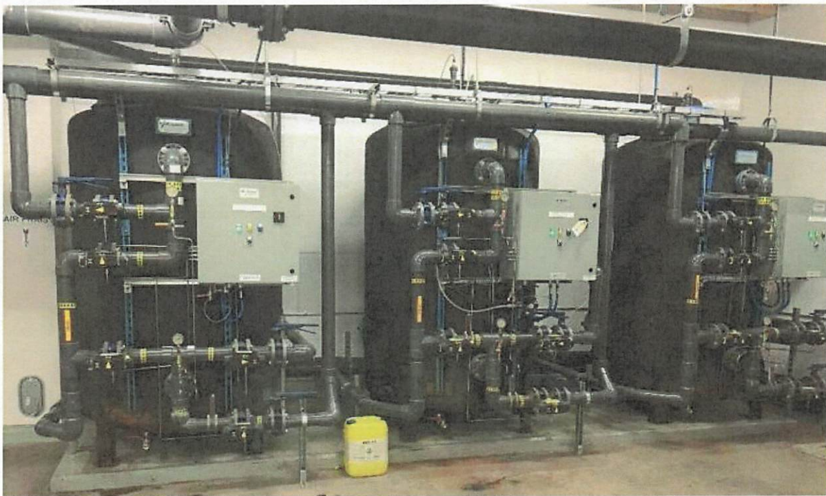
Figure 3-1: Three Vessel Greensand Filtration Process
