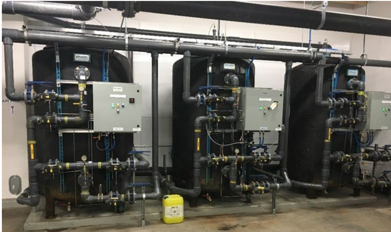
Figure 3-1: Three Vessel Greensand Filtration Process
