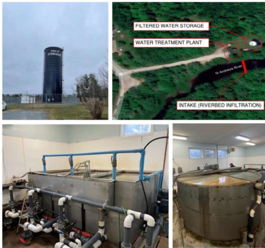
Figure 5-1: Current Water Treatment Plant on St. Andrews Street.
